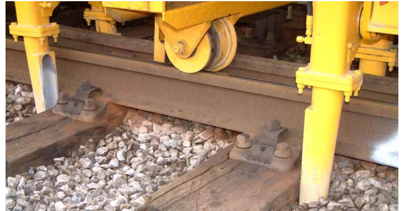
Multipurpose Stoneblower injecting stone under sleepers to lift track.
